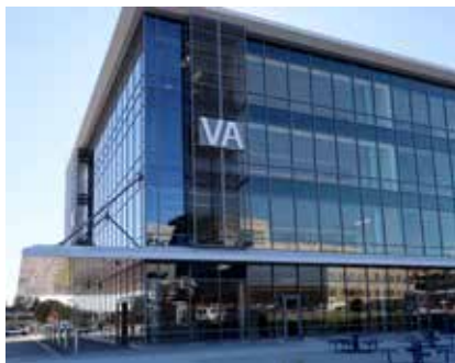
The new VA Worcester CBOC is located at 403 Belmont Street on the campus of the University of Mass. Chan Medical School.
